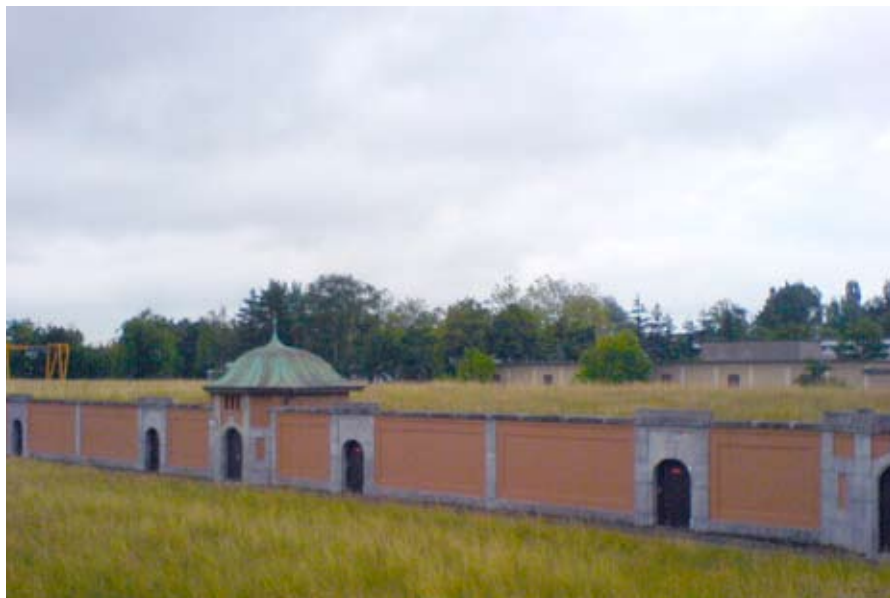
Water cleaning plant in Wollishofen (Photo by Stephan Brenneisen)
